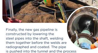
repeated until the pipe is through to the exit shaft.
