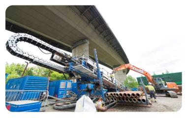
The construction of the launch shaft for the micro tunneling works has started, as has the welding of the pipeline which will be inserted during the HDD operation.
