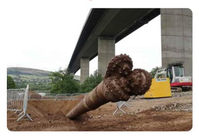
Meanwhile in Old Kilpatrick, another trenchless technique was used when we auger-bored below the existing steel gas pipeline and concrete water main within Lusset Park. Two large pits were made, the auger put in place on a set of rails and each pipe length lowered and welded before being pushed behind the auger which drills out the soil.
