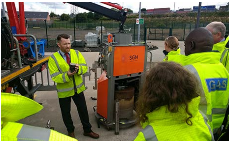
Innovation Delivery Manager Ryan Smith demonstrates iCore which reduces the size of our excavations minimising the impact of our works.
