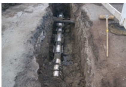
This picture shows a 4" ductile iron gas main operating at pressures between 75mbar – 2bar. This gas main has multiple temporary repairs inflicted through continuing severe corrosion. In this instance, the gas main was decommissioned due to its poor deteriorating condition.
