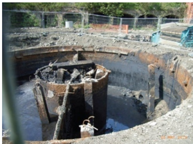
Below-ground tar tank on a former gasworks
