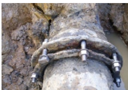
This picture shows a 12" ductile iron gas main suffering with severe joint corrosion. As can be seen the joint ring and bolts have completely corroded away. New bolts have been installed as a temporary repair measure.
