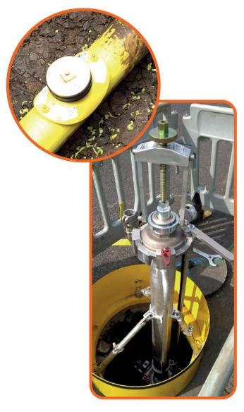
This would mean our projected asset life where squeeze off has been applied is reduced to a maximum of 45 years and where rapid cracking is present much less. Therefore, it was identified that an alternative solution to PE squeeze off should be developed which will allow for flowstopping to be carried out without causing damage and reducing the integrity and life of the asset.
