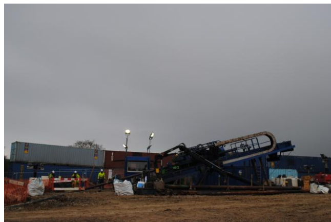
Image 11; Innovation in action. Part of the directional drilling operation under the Solent to renew and secure the gas supply to Isle of Wight commissioned in 2012.
