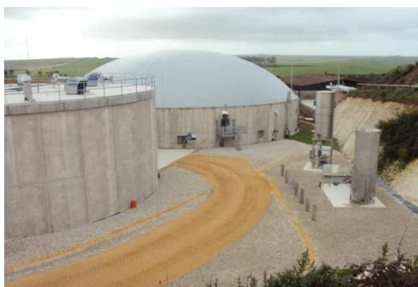
Image 8: Anaerobic digester tanks at Poundbury
