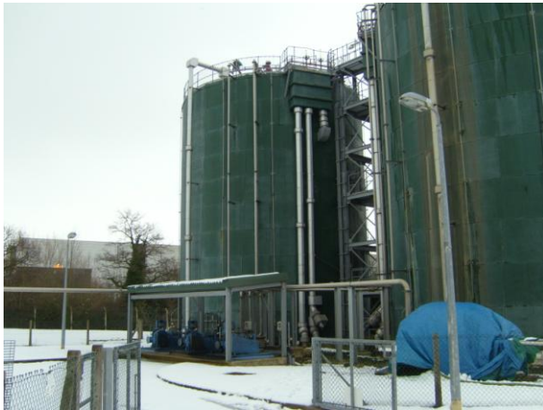
Image 6; Anaerobic digesters at UK's first biomethane plant in Didcot.
