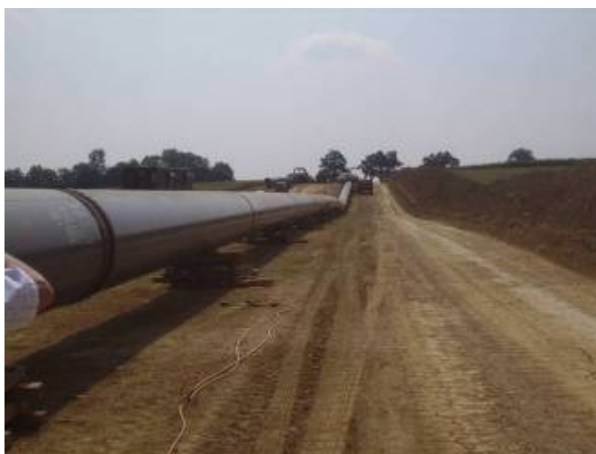
Image 6; Pipelaying as part of a major project
