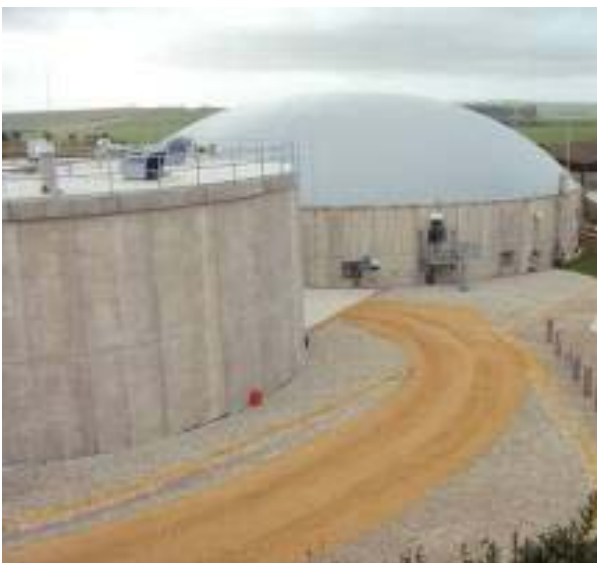
Image 8; Anaerobic digester tanks at Poundbury
