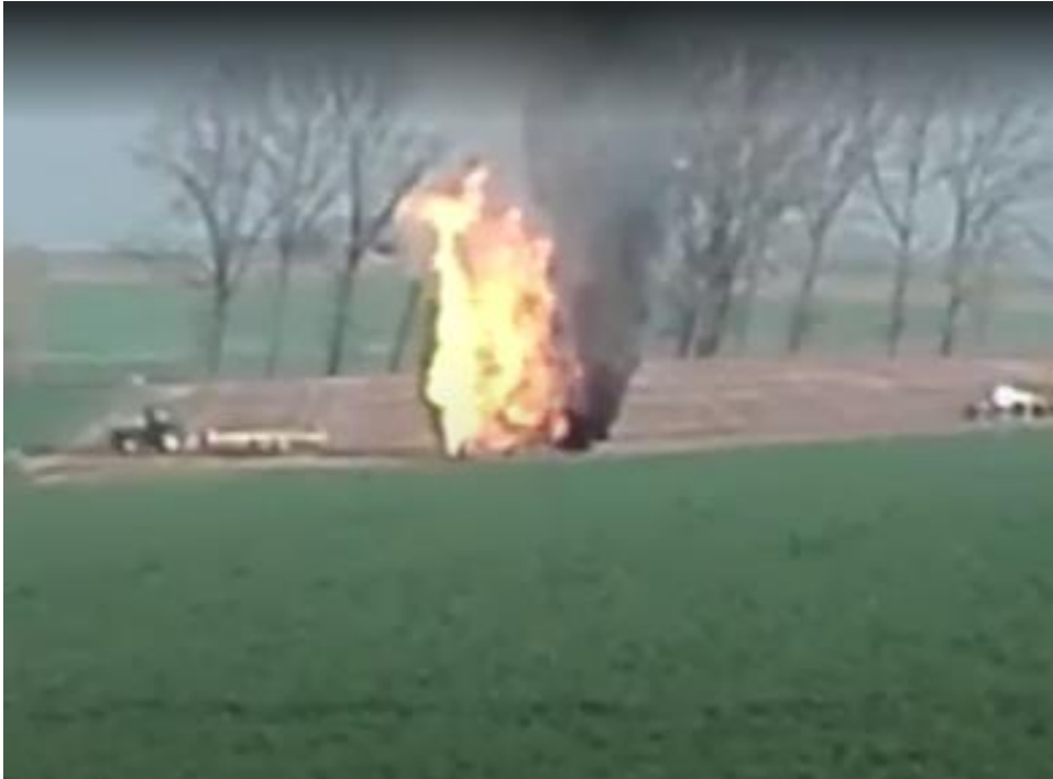
Figure 11 Pipeline fire involving hydrogen release during trenching [10]
