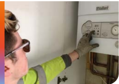
Hydrogen fuel cell technology is continually advancing for HGV vehicles. The future of gas boilers is shown here with a boiler conversion from natural gas to hydrogen.
