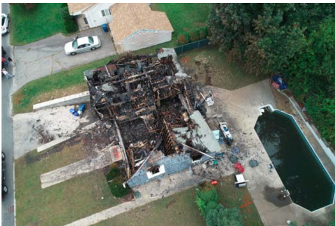
Figure 18: Aerial views of 2 homes impacted by the over-pressurisation incident in Massachusetts. The event caused significant fire damage (Left) and a fatality after a chimney collapsed on a vehicle parked in the driveway (Right).
