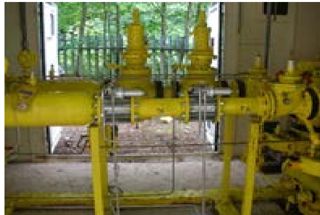
Figure 17: West Kilbride - before and after installation of maintenance-free, OxFlow Regulators
