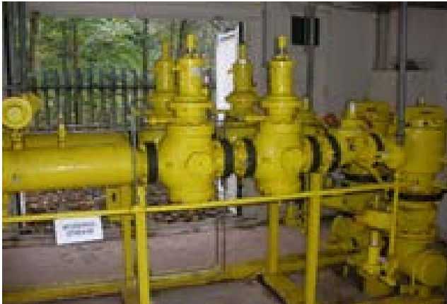
Figure 17: West Kilbride - before and after installation of maintenance-free, OxFlow Regulators
