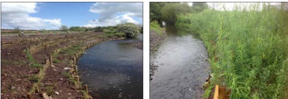
Figure 7: Example of Newly Installed Terraced Willow Spiling ( Images property of SEPA – Scottish Environment Protection Agency )
