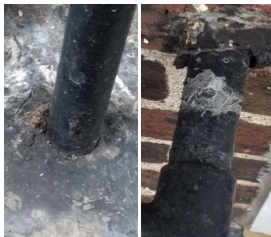
Figure 21. Risers requiring replacement
