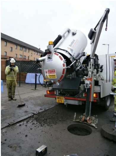
Figure 7: Coring operation
