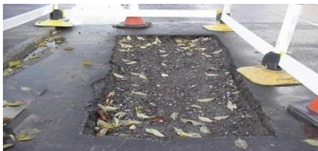
Figure 6: Guarded excavation
