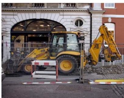
Figure 5: Excavation in progress
