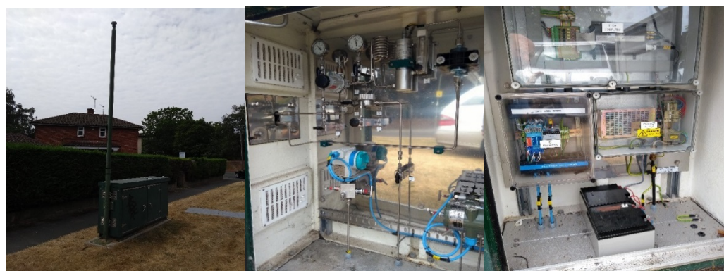
Figure 16: Inter LDZ Site - Kiosk, Gas PT, Flow Equipment and Comms Equipment
