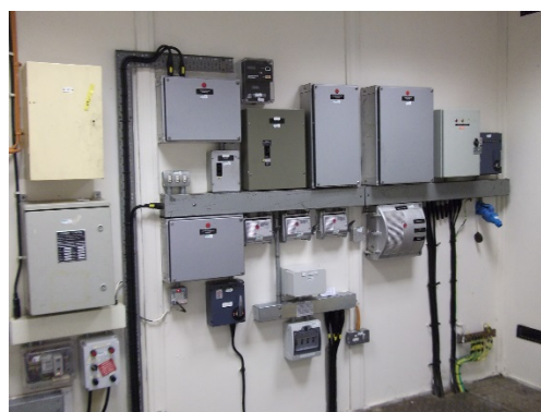
Figure 17: Asbestos containing distribution kit at Soutra Offtake
