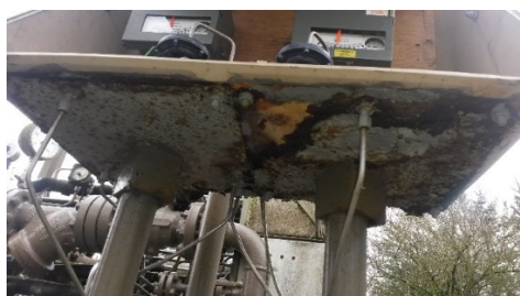
Figure 19: Corroded Comms Kiosk and Up and Over Kiosk
