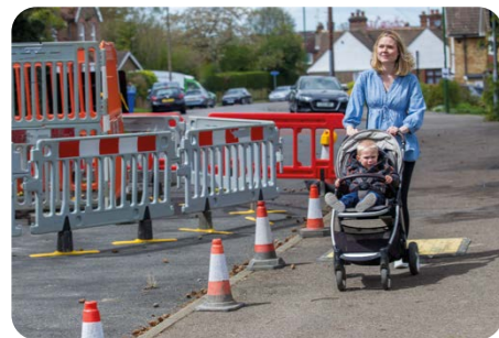
Ensuring site safety for all pedestrians and cyclists.
