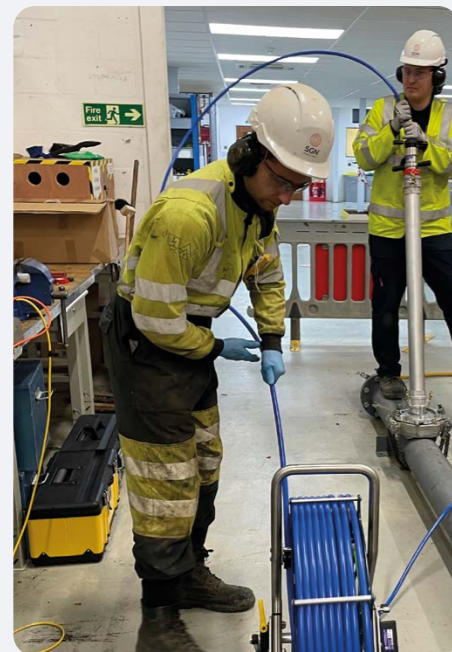
↑ Improving safety for our employees and the public.
