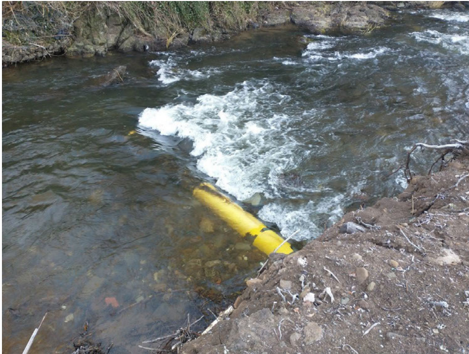
Figure 7: Exposed section of IP pipe crossing River Dighty.
