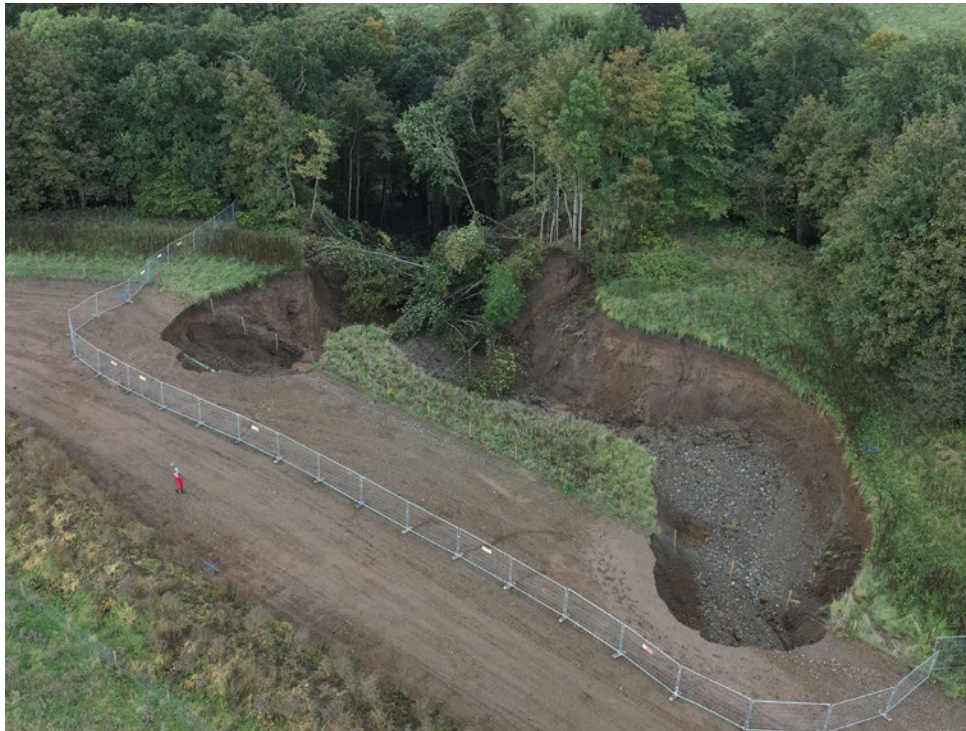
Figure 6: Scale of damage caused by washout on Pitcairngreen to Huntingtower pipeline.
