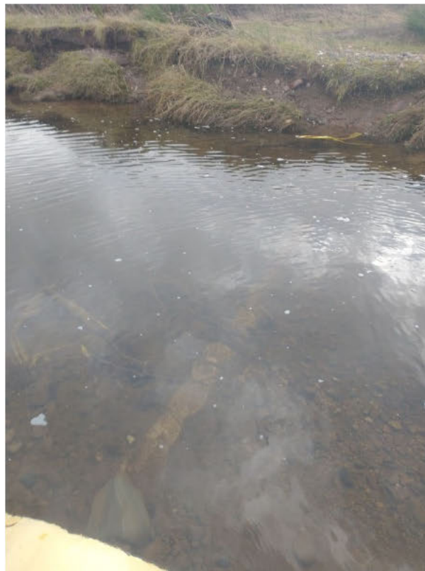
Figure 8: Exposed sections of pipe covered in flood water.
