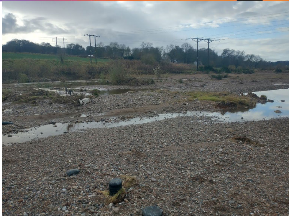
Figure 9: Extent of washout on landscape, with stopalls for original diversion in foreground.
