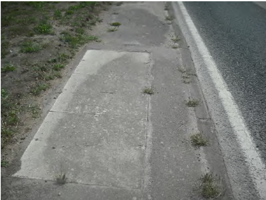
British Telecom route works evidence in carriage way, footpath, and verge.
