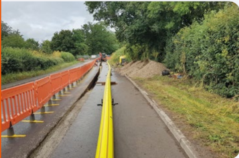
Mains replacement programme – we’re replacing our old metal gas pipes with new PE pipes.
