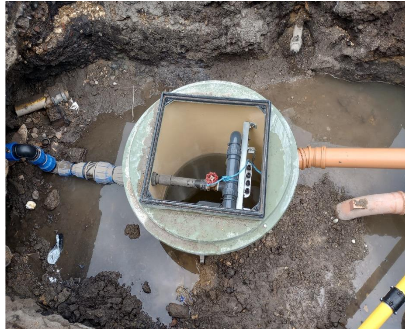
Installation of new pump
