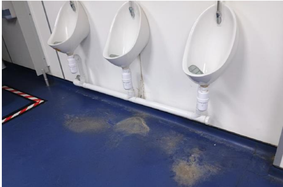
Toilet facilities before
