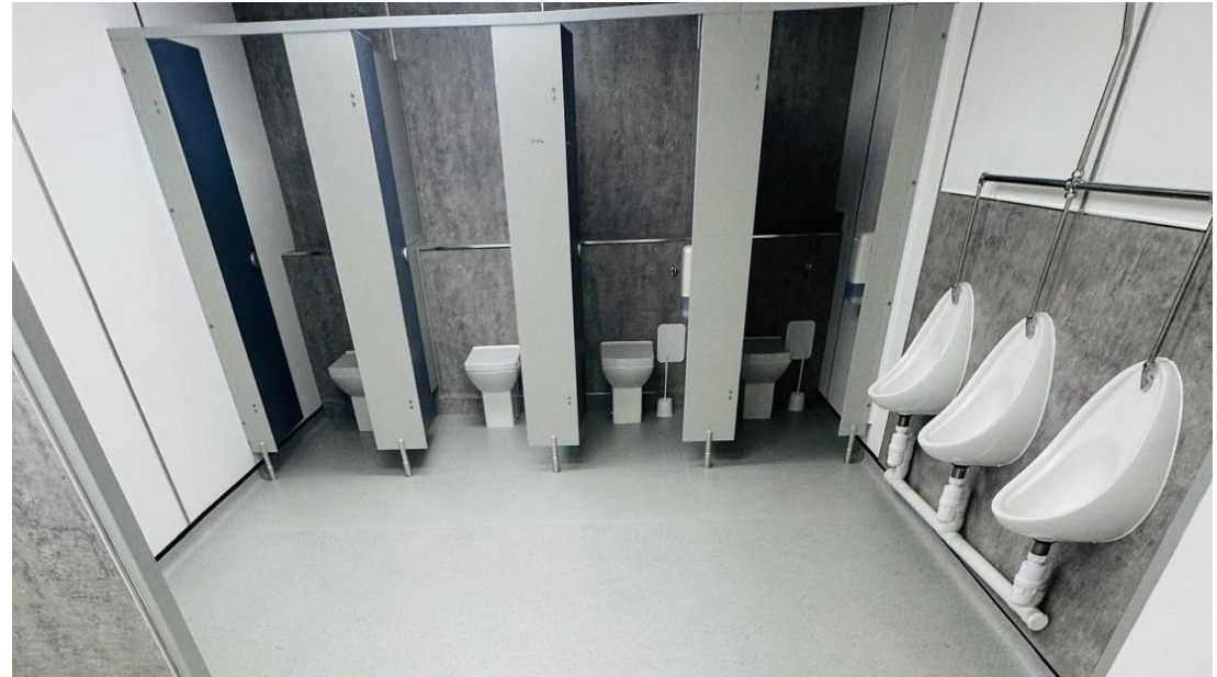
Toilet facilities after
