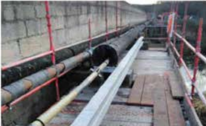
Figure 7: River Avon bridge crossing construction.
