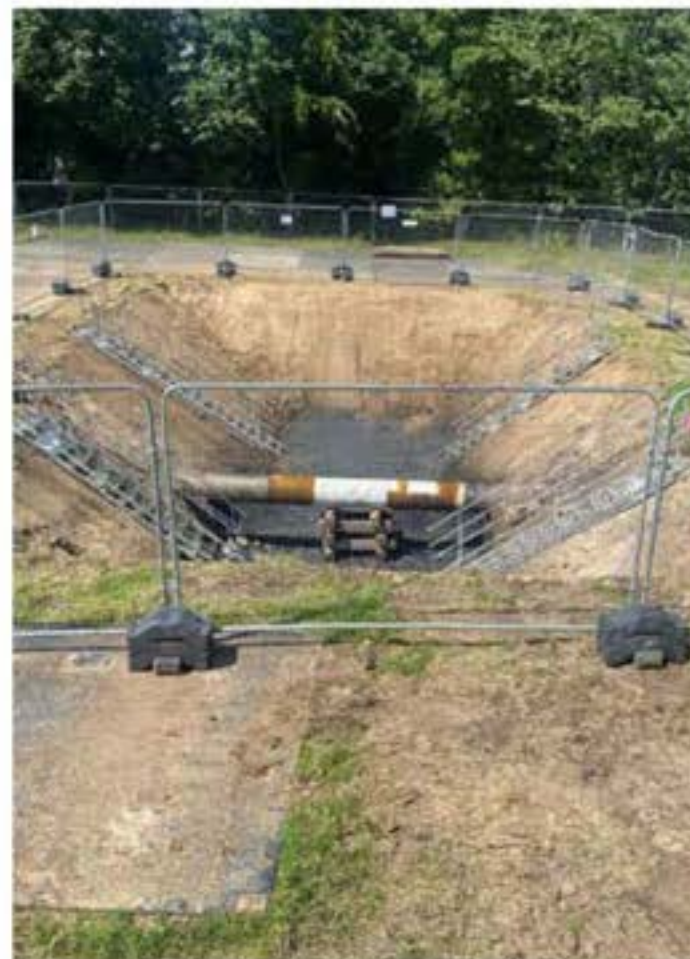
Figure 48: Excavation after completion of NDT.
