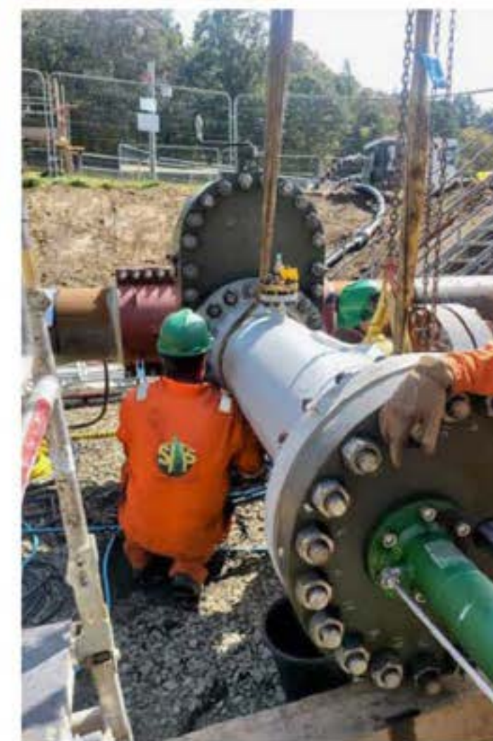
Figure 65: BISEP flow stopping tool.
