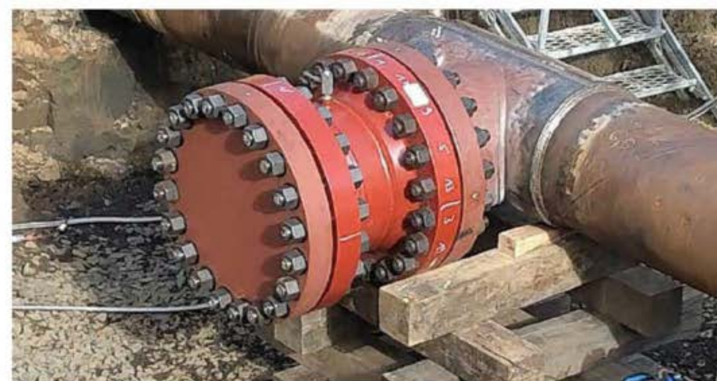
Figure 60: Set-on fitting final blank.
