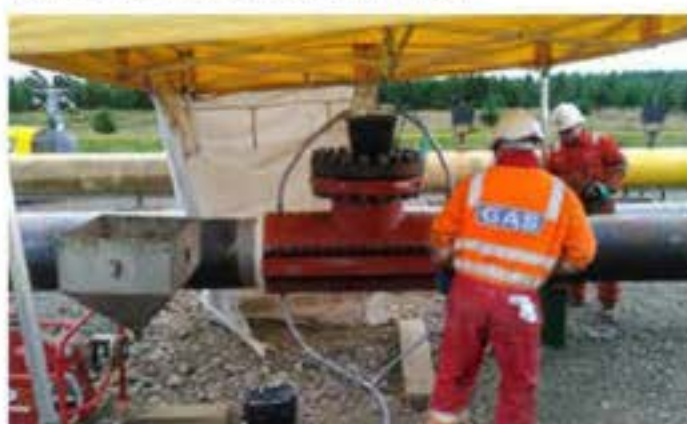
Figure 32: Injection of grout into vertical tee.
