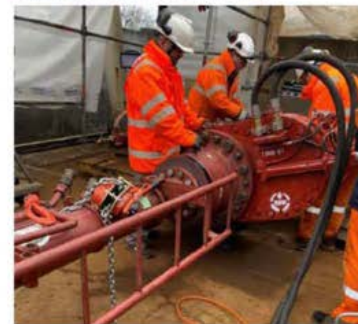
Figure 41: FAT preparation of hot tap machine.
