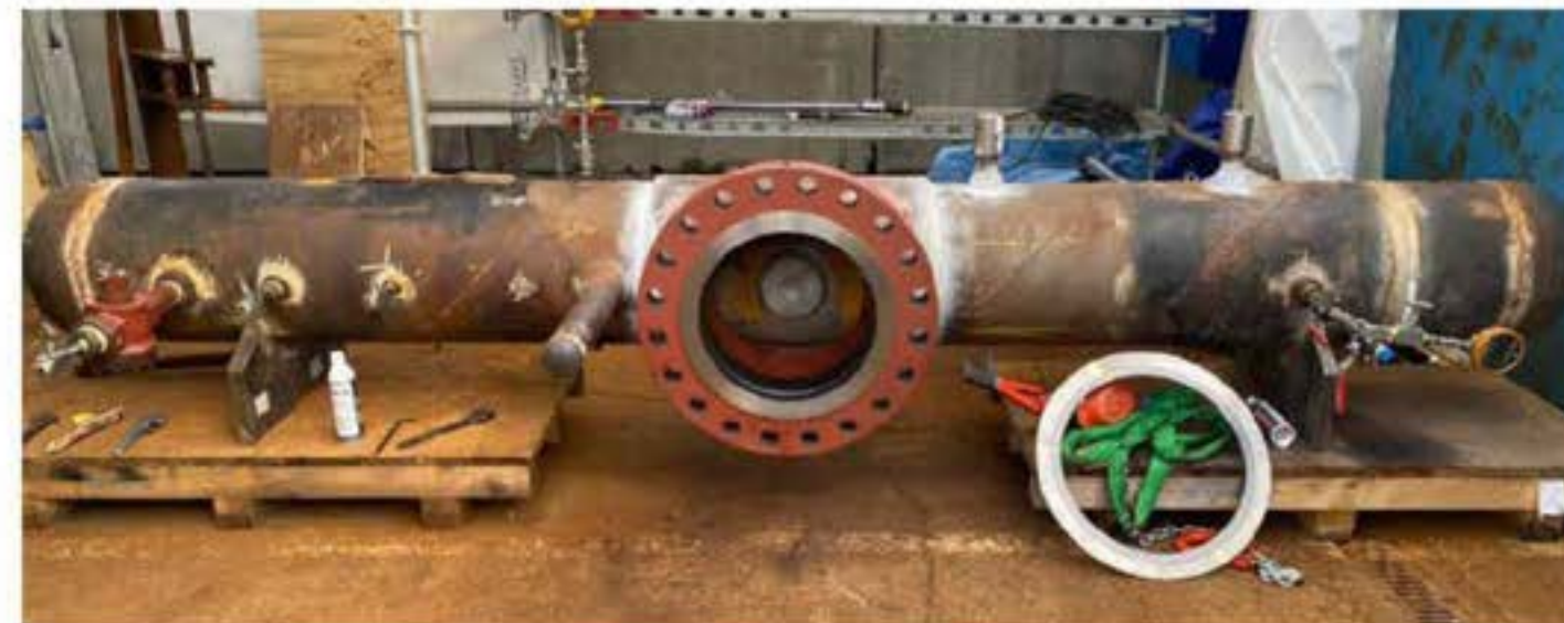
Figure 40: FAT vessel upon completion of welding.
