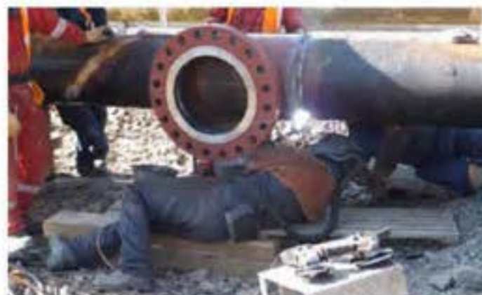
Figure 32: Injection of grout into vertical tee.
