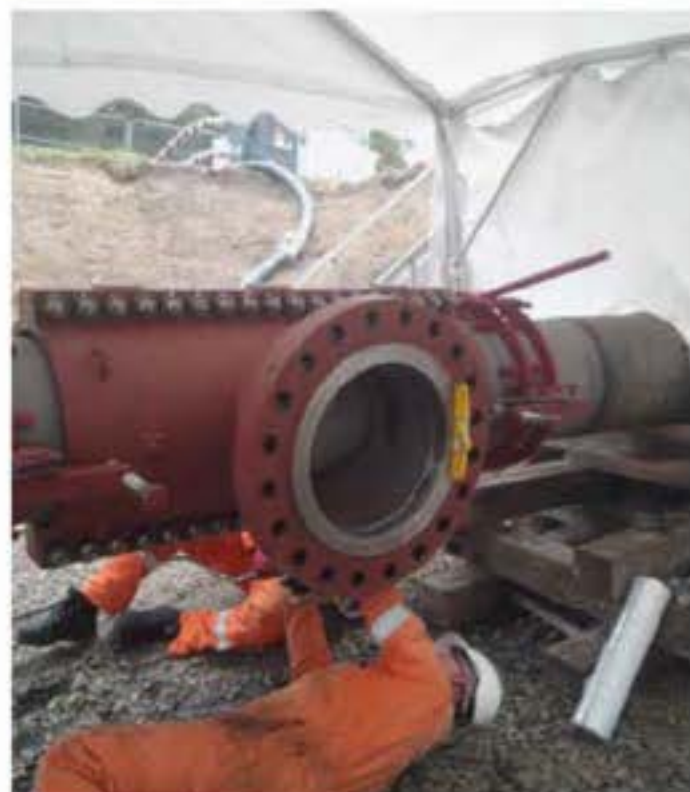
Figure 61: Grouted tee install.
