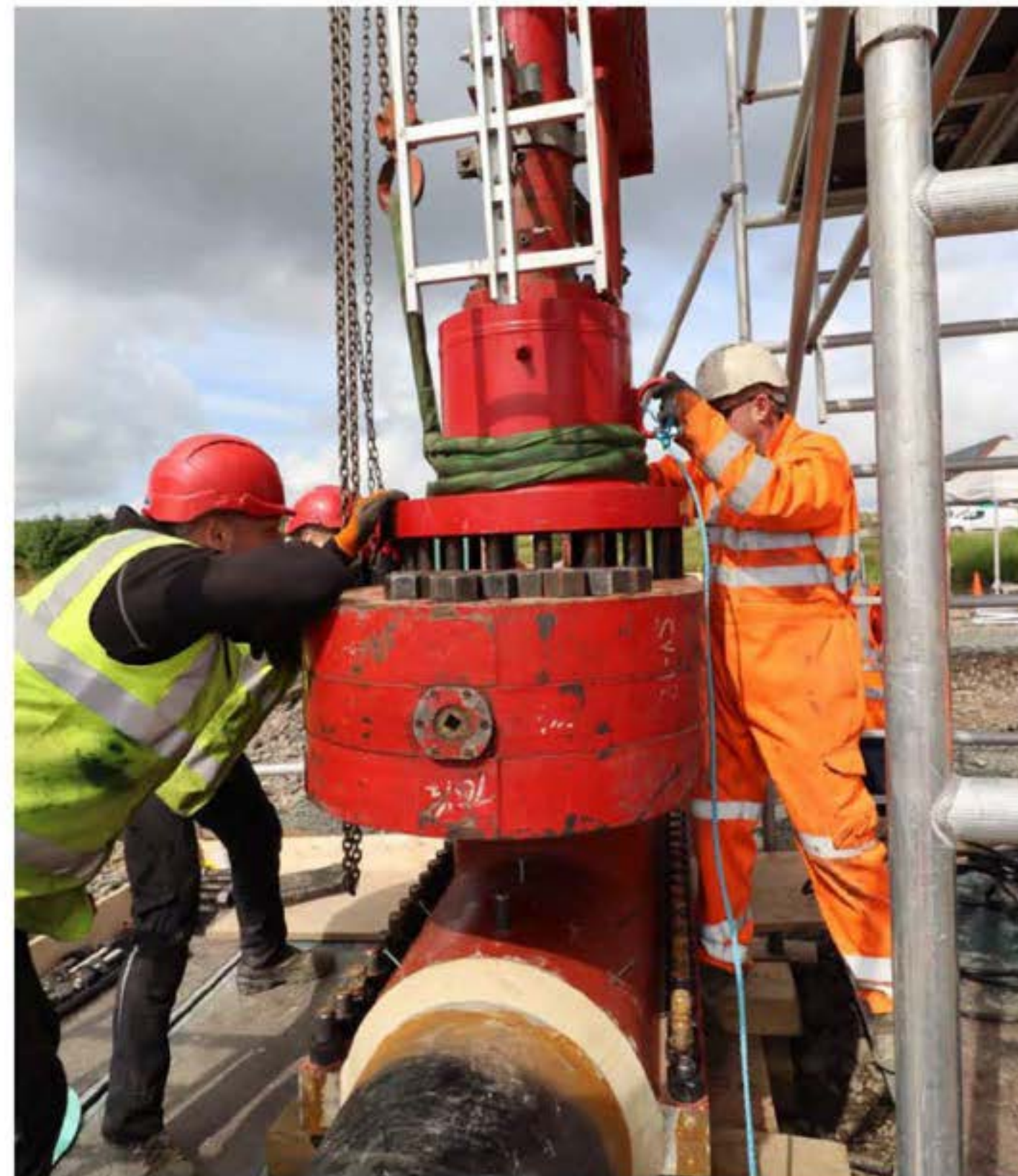
Figure 37: Hot tapping qualification.
