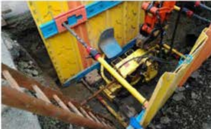
Figure 6: Gateway 7 moiling pit.
