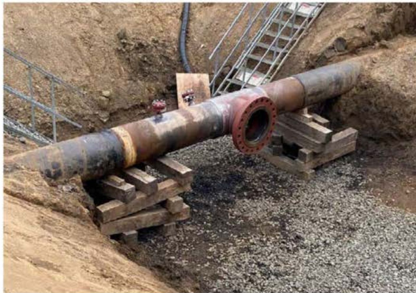
Figure 53: Split tee and set-on fittings successfully welded onto a live hydrogen pipeline.
