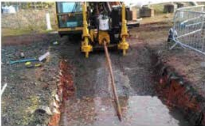
Figure 8: HDD exit INEOS FPS site.
