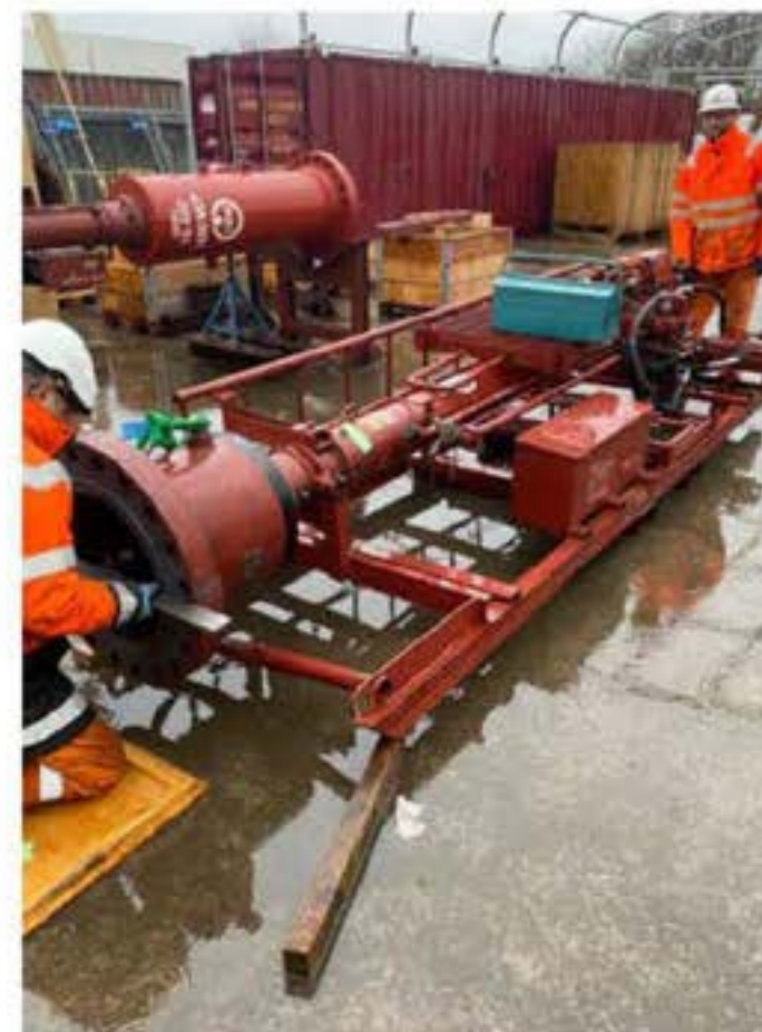
Figure 34: Tapping machine, sandwich valve and cutter head.
