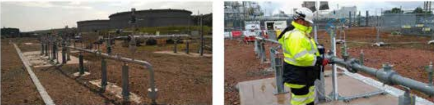
Figure 11: Hydrogen entry unit.
