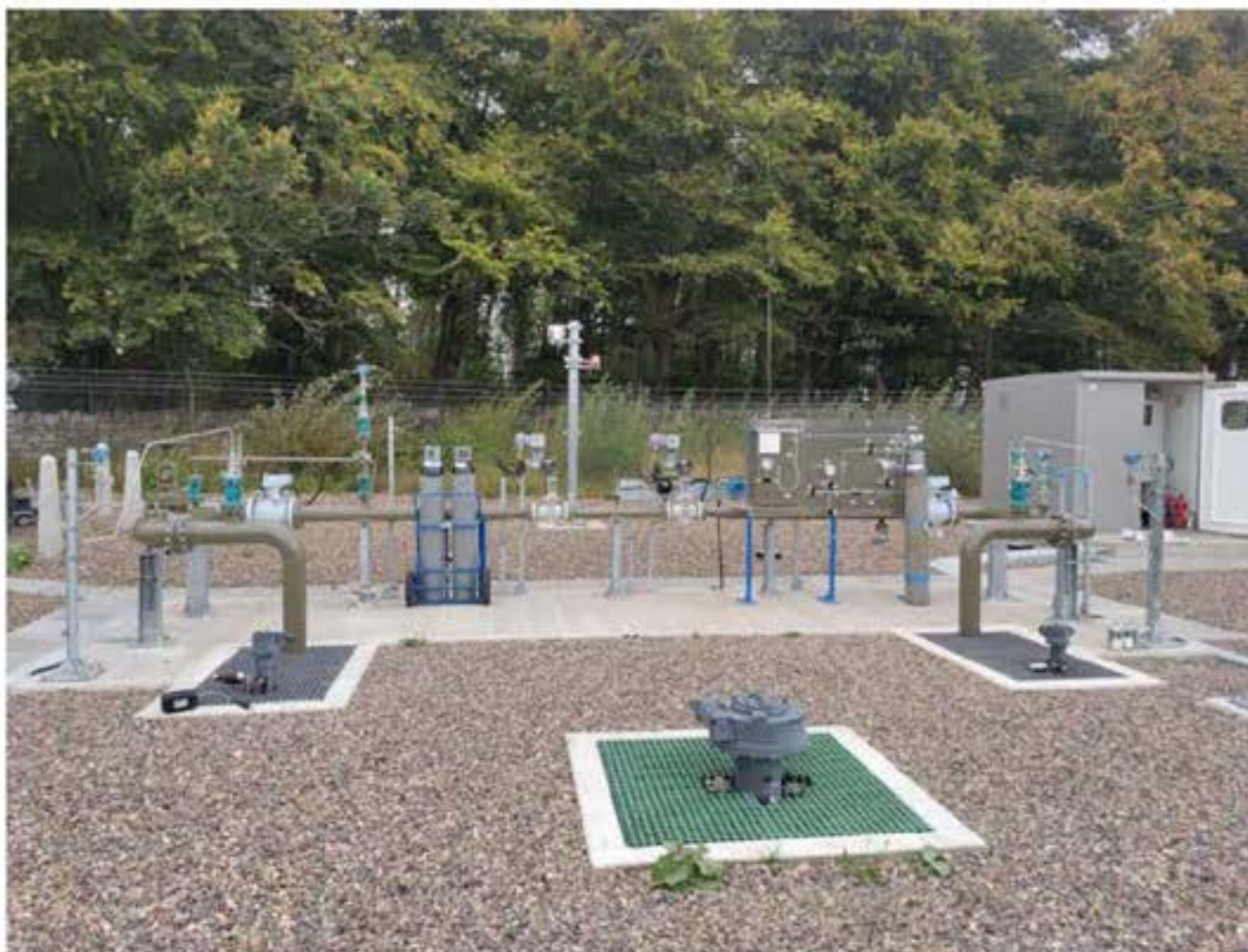
Figure 12: Newton block valve by-pass.
