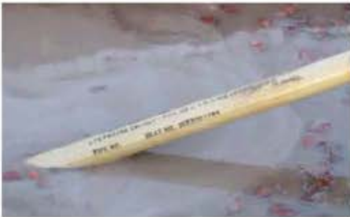
Figure 9: Pipe string on exit.
