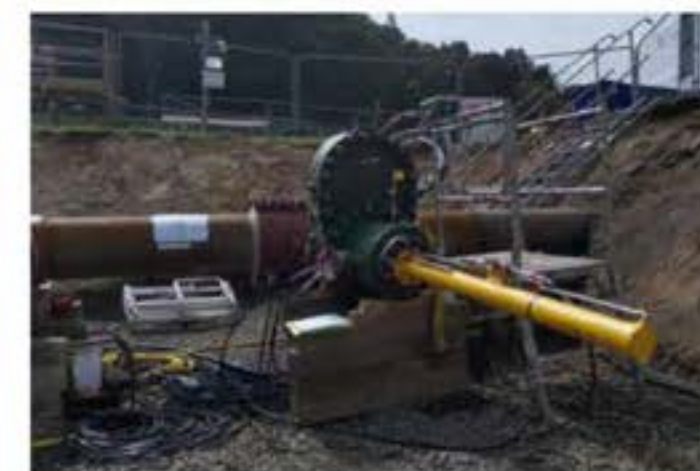
Figure 64: Swarf management tool.
