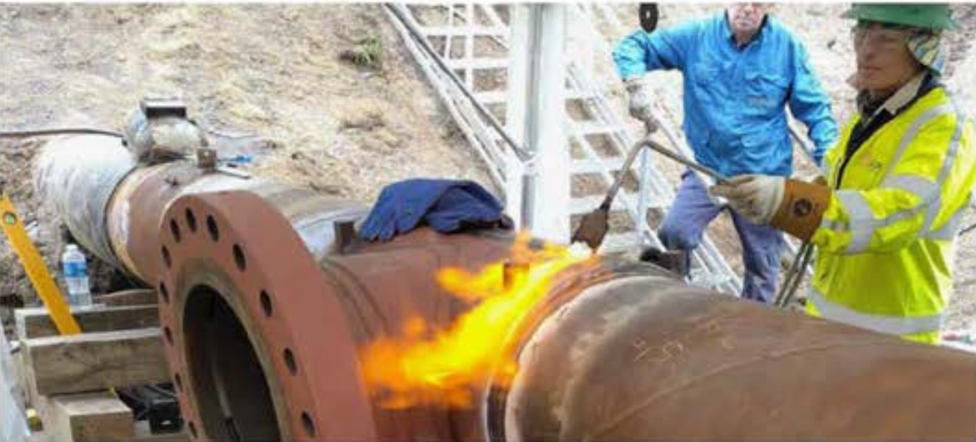
Figure 27: Pre-heat application for split tee welding.
