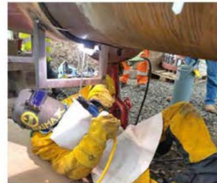
Figure 50: Longitudinal seam welding.
