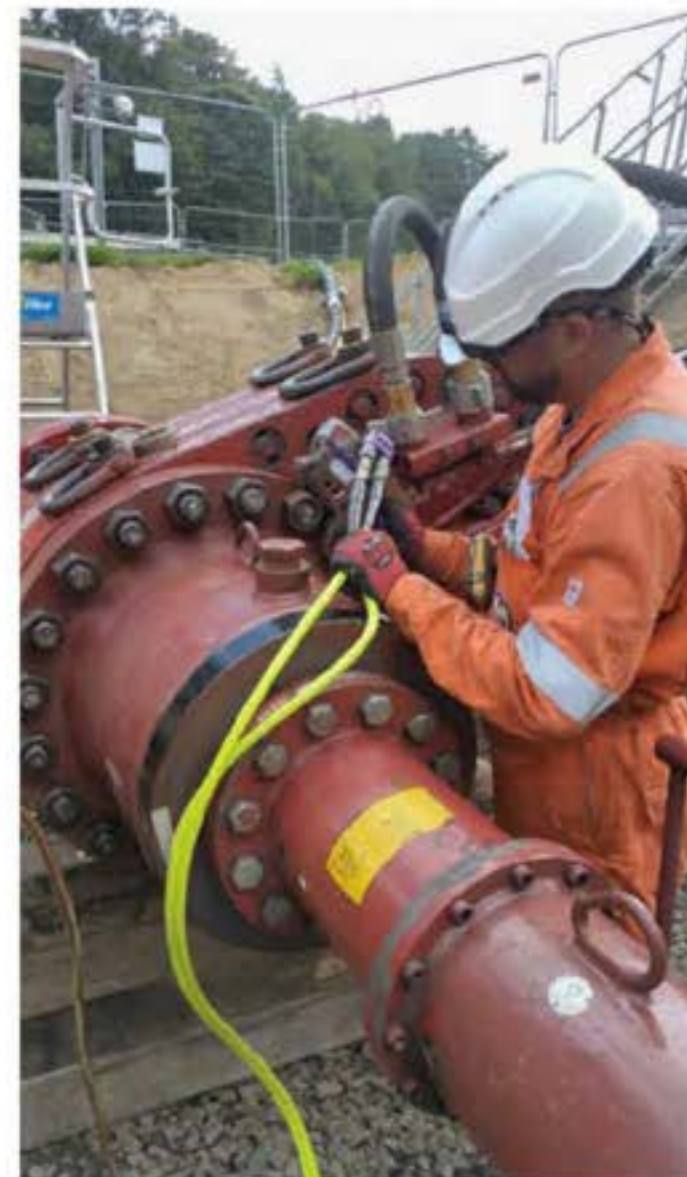
Figure 55: Fitting the tapping machine to the sandwich valve.
