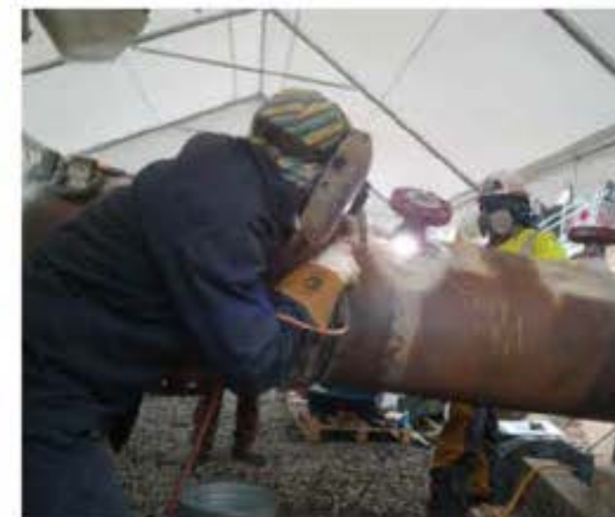
Figure 52: Set-on fitting welding.
