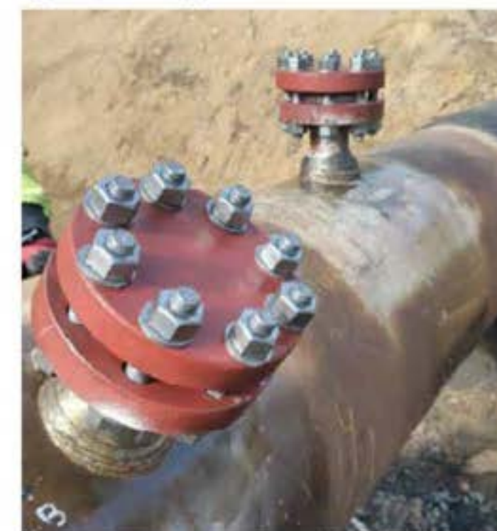
Figure 60: Set-on fitting final blank.
