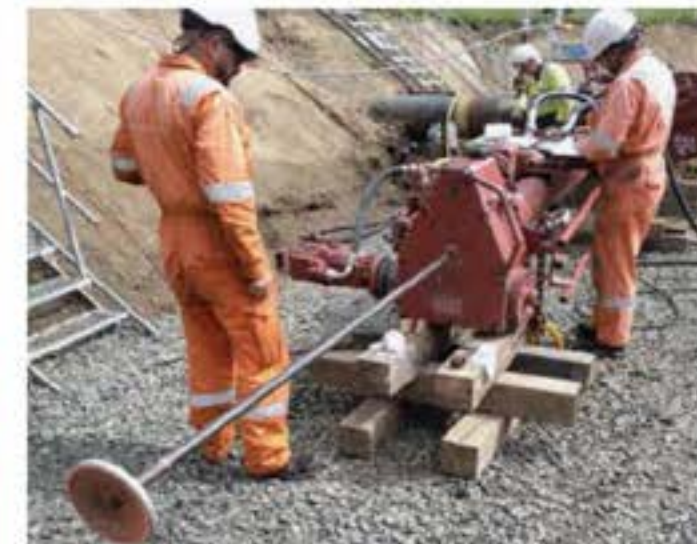
Figure 57: Hot tapping of set-on fittings.
