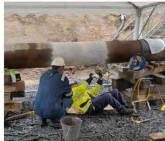
Figure 49: MPI on fitting area.
