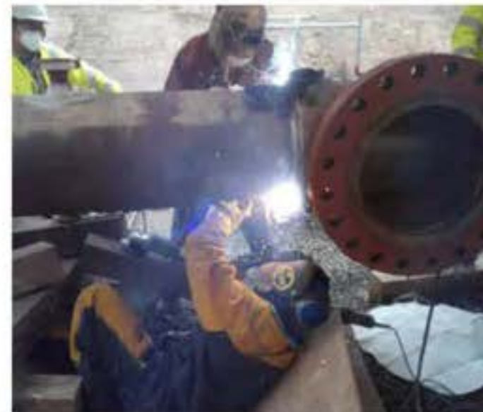
Figure 51: Circumferential welding.
