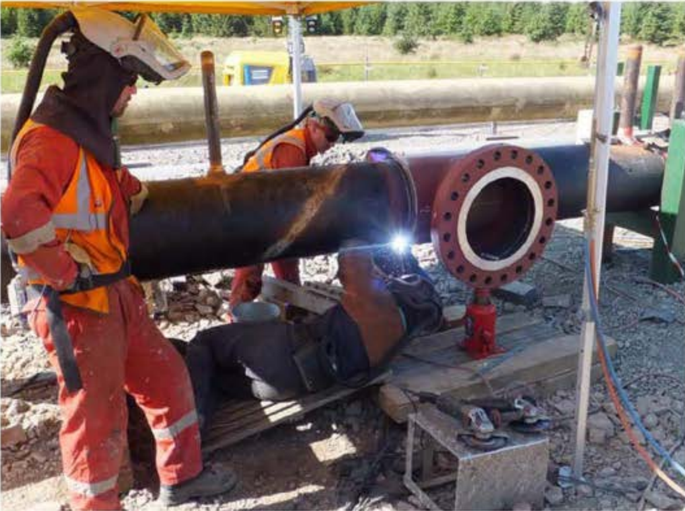
Figure 22: Live welding.
