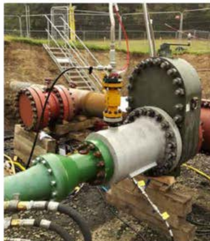
Figure 62: Hot tapping of grouted tee.
