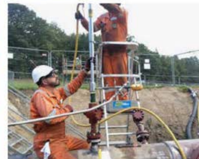
Figure 57: Hot tapping of set-on fittings.
