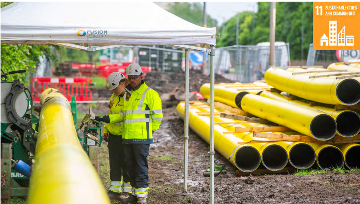
Historical pipeline washout data provides insight into the operational and financial impacts of extreme weather on our network
