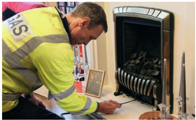
Local space heater test
